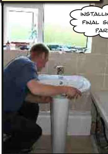
NEW BASIN INSTALLED...
